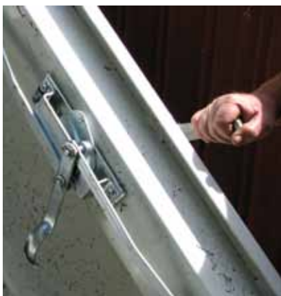
The steel door is installed with a gas spring cylinder.
