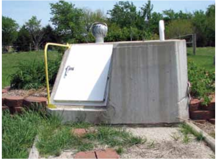
This storm shelter meets and exceeds FEMA requirements.
