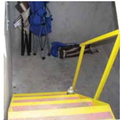
Storm shelters have non skid steel stairs and can have hand rails installed.
